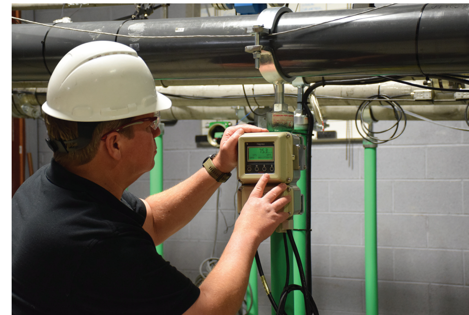
▲ Figure 4: Particulates and dissolved solids can affect mag meter performance. Abrasive slurries moving at high velocity can wear away lining material; high concentrations of solids can generate electronic “noise,” which limits the usefulness of an instrument that uses electromagnetism to read flow.
